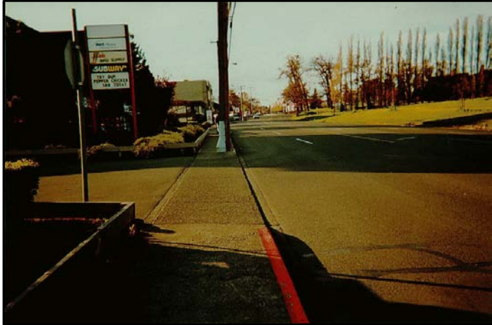
Monolithic sidewalks, west side of West Saanich Road. Note the lack of boulevard and utility pole blocking pedestrian flow.
