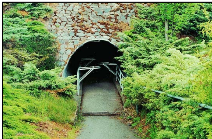
Highway 17 pedestrian underpass requires upgrading.
