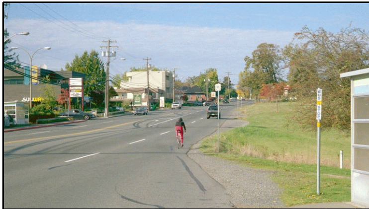
West Saanich Road looking North towards Fireside Grill Restaurant. Note lack of bicycle lanes and pedestrian facilities.
